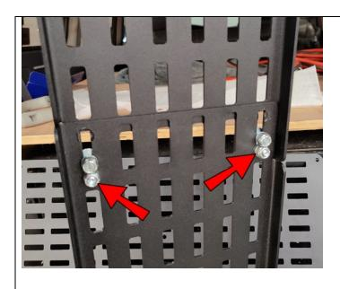
This next step is VERY important! If the ends aren't butted tightly against each other before tightening, it will cause the panels to sag when installed.
