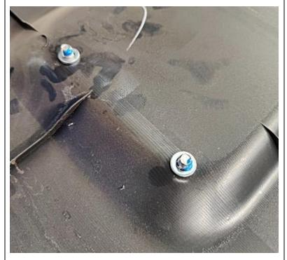
Put some threadlocker on each of the bolts then secure with M6 Nuts and tighten.
